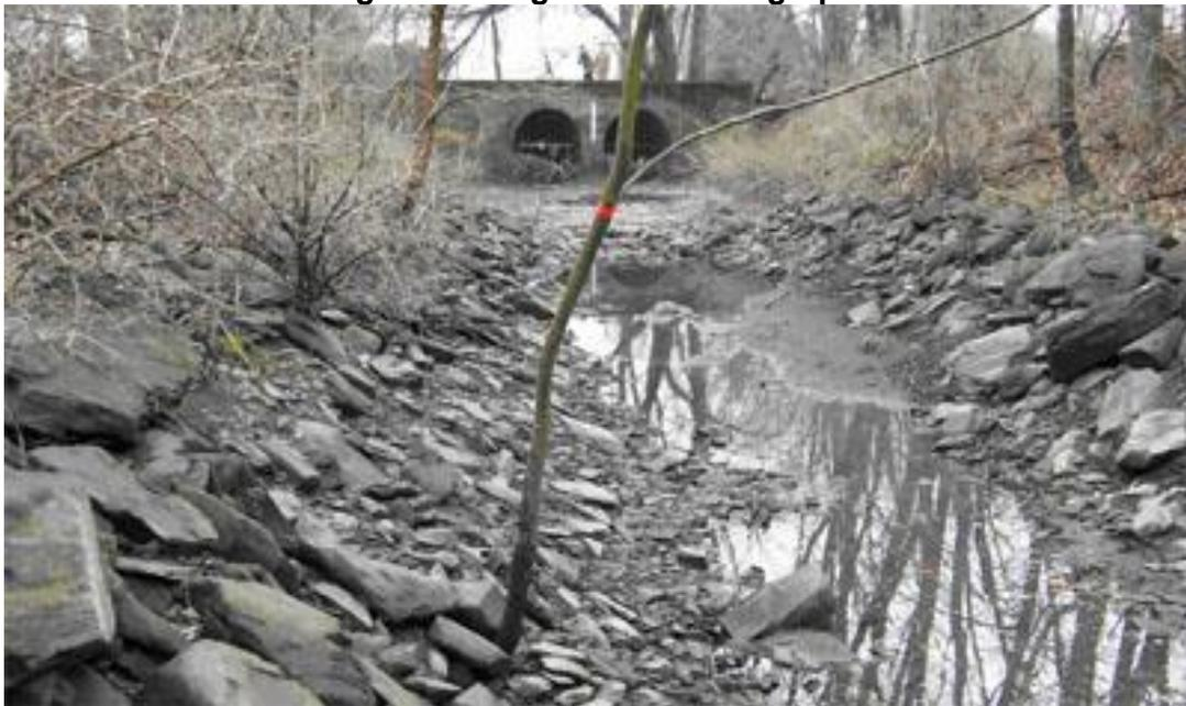
Portions of Segment 1 were excavated and replaced with riprap in an effort to remove the contamination and stabilize the banks. The banks above the riprap, which did not undergo excavation, contain the highest concentrations of COCs. Bioremediation is a solution as to how the contamination on steeply sloping banks and in the channel could be addressed without removing vegetation or performing costly and ineffective excavation.
